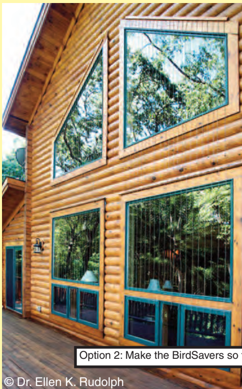
Photo above: Volunteers at the Chincoteague National Wildlife Refuge installed Acopian BirdSavers on windows to prevent bird mortality. Photo credit: USFWS
