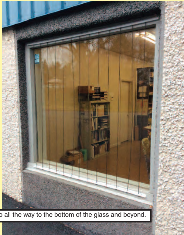
Photo above: Volunteers at the Chincoteague National Wildlife Refuge installed Acopian BirdSavers on windows to prevent bird mortality. Photo credit: USFWS
