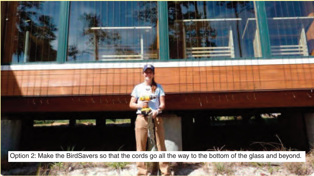
Photo above: Volunteers at the Chincoteague National Wildlife Refuge installed Acopian BirdSavers on windows to prevent bird mortality. Photo credit: USFWS
